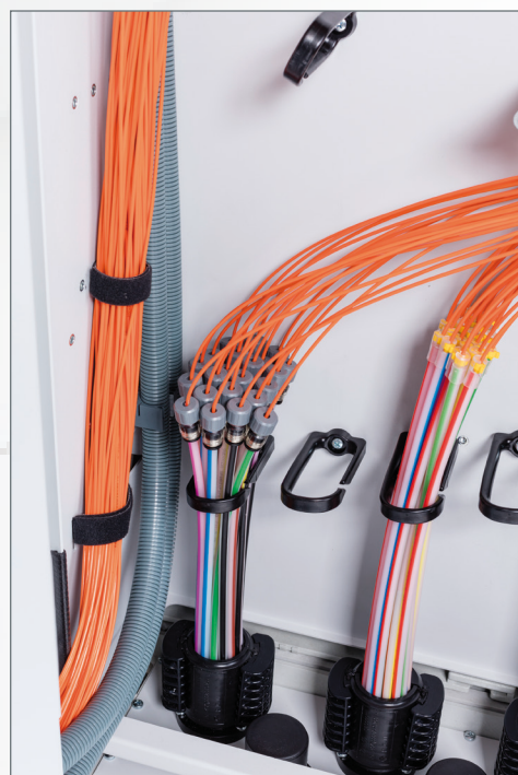
The innovative tube insertion system of the new 2Line NVT
