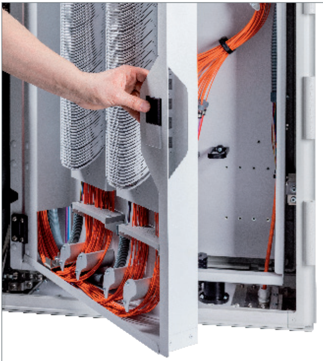
Access to the tube area via a stable hinged door
